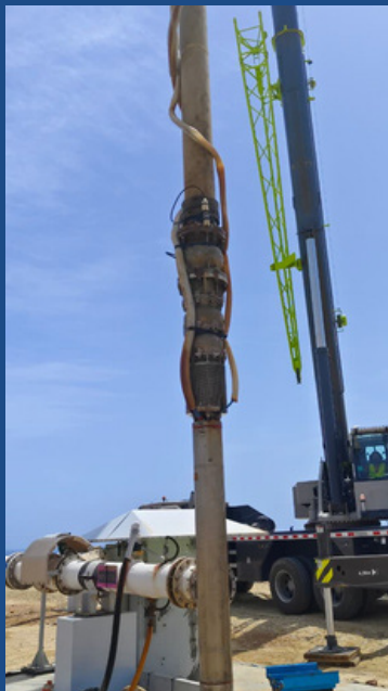
FIGURE 2 - PUMP DETAILED INSPECTION: A) PUMP BEING REMOVED FOR DETAILED INSPECTION B) INSULATION RESISTANCE TEST SHOWING 0 MOHM
